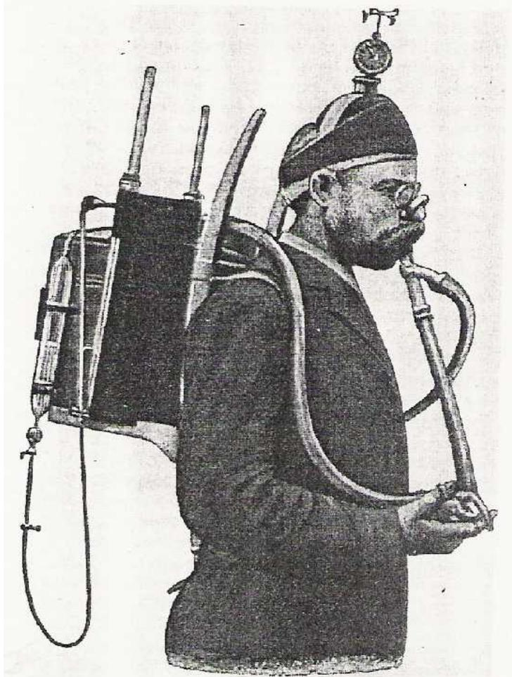
Fig. 3. Adolf Loewy (1862–1936) wearing the transportable Gasuhr (transportable gas measuring device) invented by Zuntz for field studies and an anemometer to measure air velocity at the top of his head.
